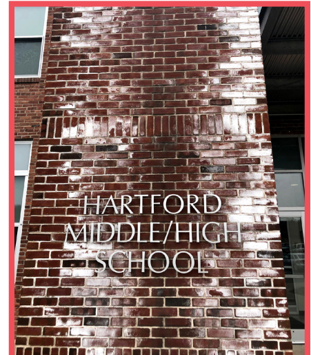
Brickwork at the Middle/High School entrance is need of repair.
